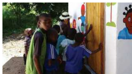
Renovation waterworks and bathrooms in elementary school
